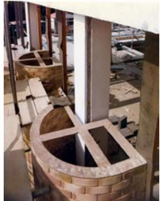
**AFTER:** the concrete pillar becomes merely one amongst many pieces of physical 'kit' within the ample stomach of the column of the 'Ordine Robotico'. A plywood template uses the structural frame as a trammell to guide the bricklayer upwards.
