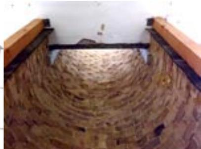
The over-cladding in wood and brick could be made by any builder. It was cheap, durable and maintenance-free.
