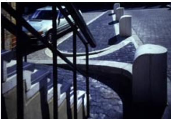
**AFTER:** Showing the new pre-cast treads and the new handrail. The new kerbs flow as does also the interlocking block paving. Iconically they celebrate Okeanos.
