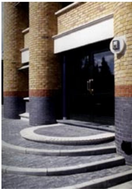
Specially pre-cast curved steps with deep anti-freezing grooves and extra-solid cantilever step-nosings.
