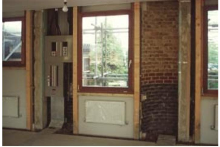
**AFTER:** The servicing, and the columns, are placed outside the lettable area. The brick drums were insulated internally, by foam-filled duct doors. Enough glass means small radiators. Simple and cheap.
