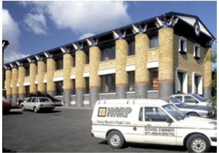
**BEFORE:** The Concrete frame of the Gatehouse was extended in steel. Steel is like the whalebone in corsetry. Why use anything so easily rusted, and melted, and so conducive of noise and heat, for anything except its enormous strength and stiffness?
