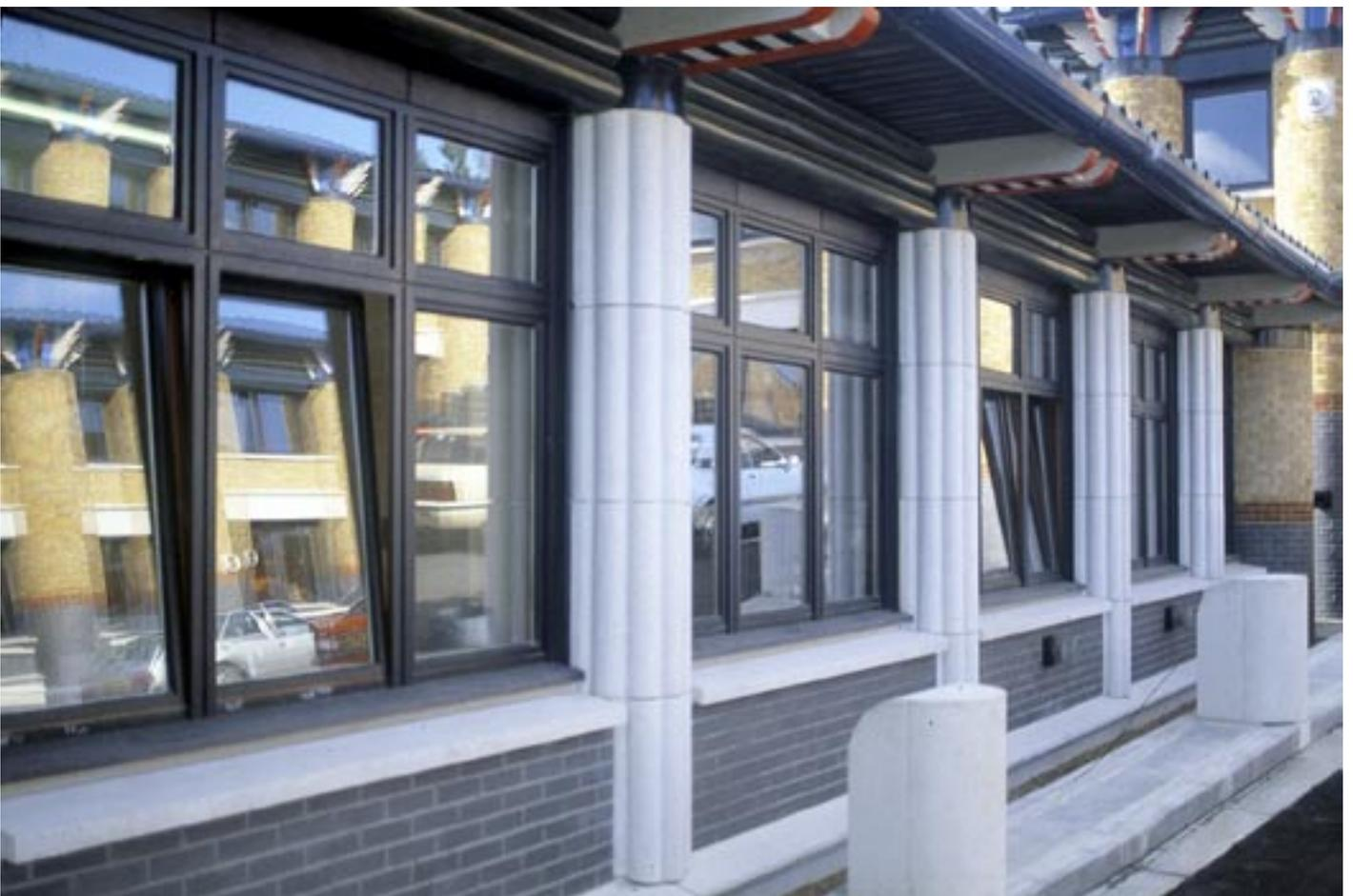
*Amplly-dimensioned stained hardwood windows, the colour of 'shadow', with a microporous finish are protected from the sun by a wide eaves. Windowframes are amongst the more iconically trivial of a building's features. They should always be unobtrusively coloured. Two 'balanced-flues' are set into their black concrete castings below the windows.*
