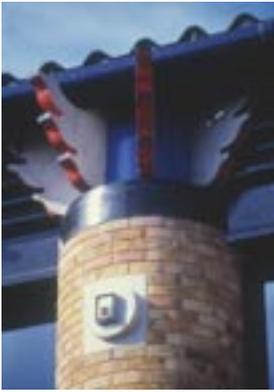
The thin skin of a Robot Column erupts with a techno-pustule. In this case it is a balanced flue.
