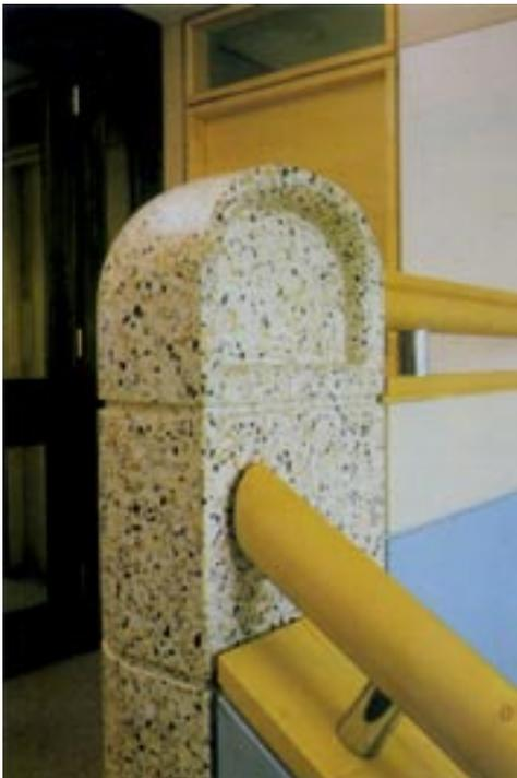
*The stairs had to be remade with a steel frame. So they could carry these lovely, solid terrazzo, newels. The mixture of marble chips was precisely specified for the firm of Diespeker to cast and polish smooth.*
